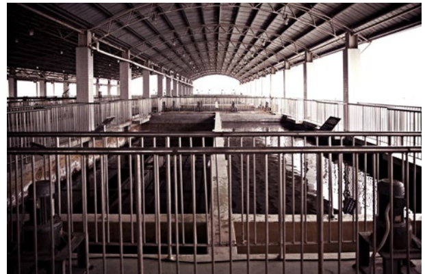
Water treatment plant at one of the factories.
